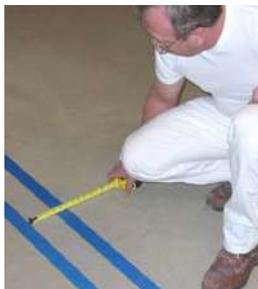
After completing four to five feet of taping (and periodically throughout the project) stop and check the width and positioning of the tape, making any minor adjustments if necessary. This will minimize lost time if any corrections need to be made.
